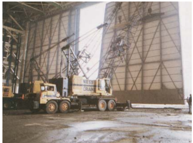
International Door installing 360' x 82' door at the world's largest building - Everett, WA.
